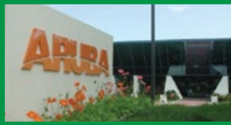
Data Center Aruba Arezzo
