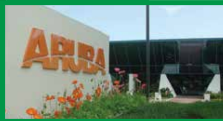
Data Center Aruba Arezzo
