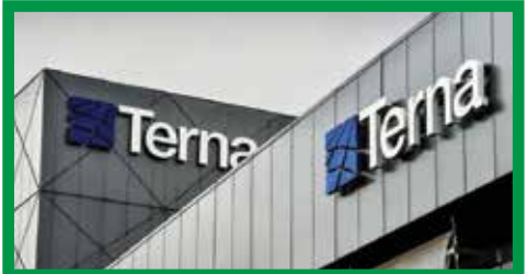
Data Center Terna Milan
