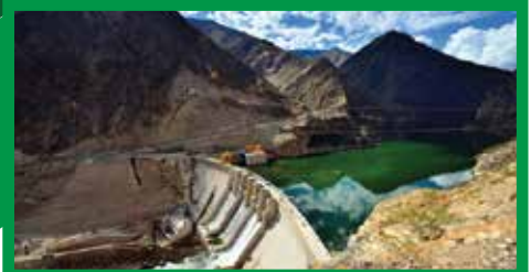
Hydroelectric Power Station Cerro De Aguila Callao
